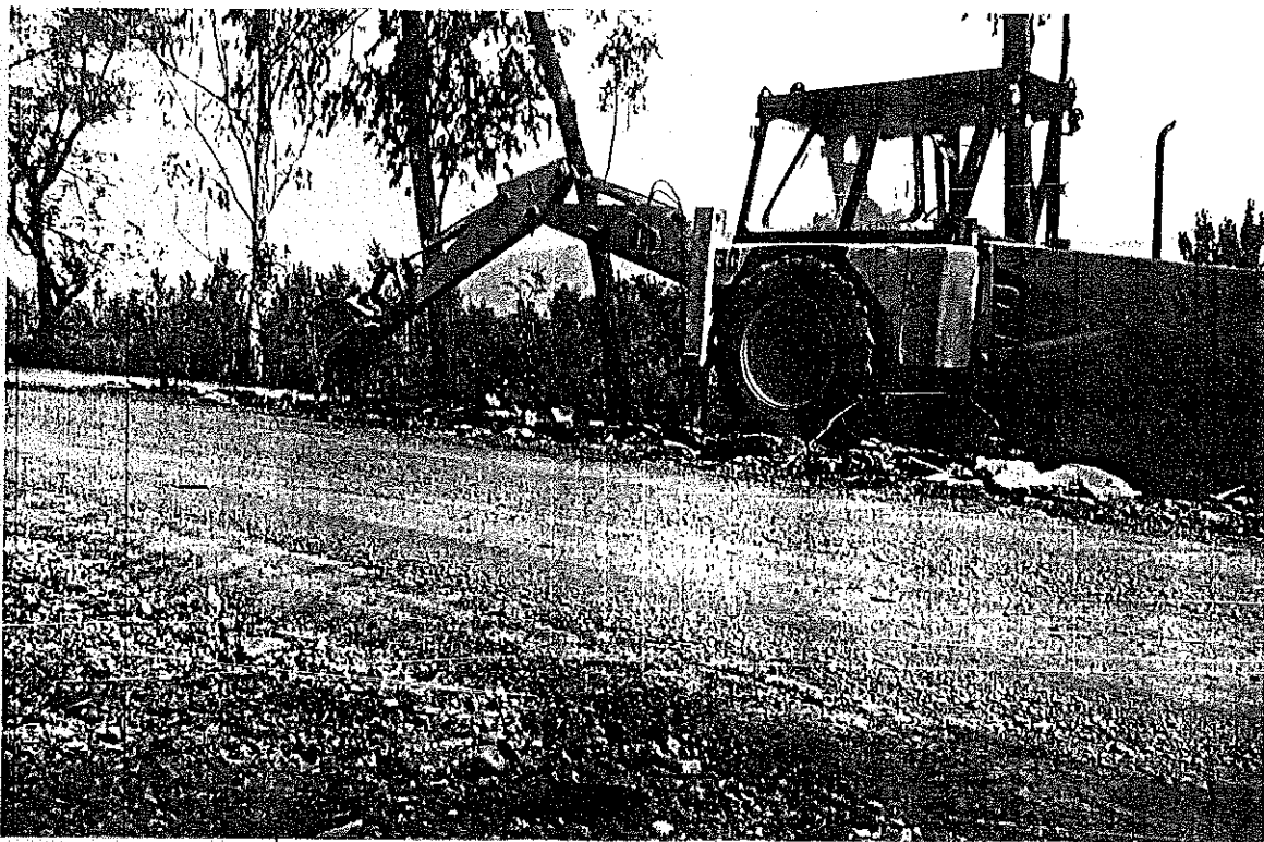
5. Pavement wearing course layer being scarified using 'un-specified' technique. The base course is prone to damage
