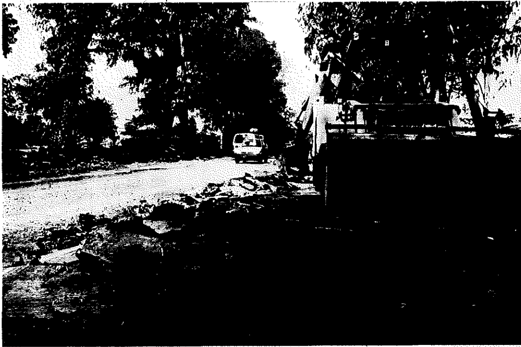
6(a). A view of scarification work. Works going on without any safety precautions
