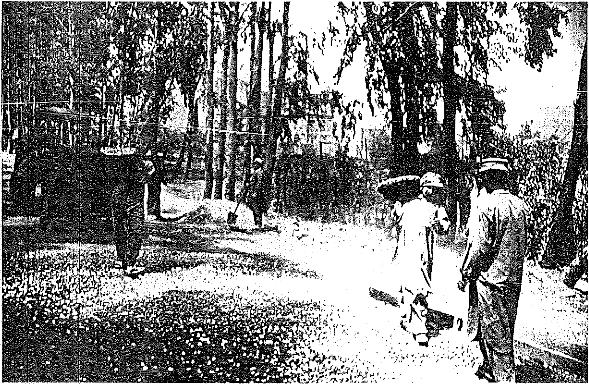
13. A view of double surface treatment works
